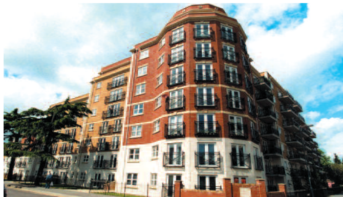
Park View - new residential complex connected to DH
